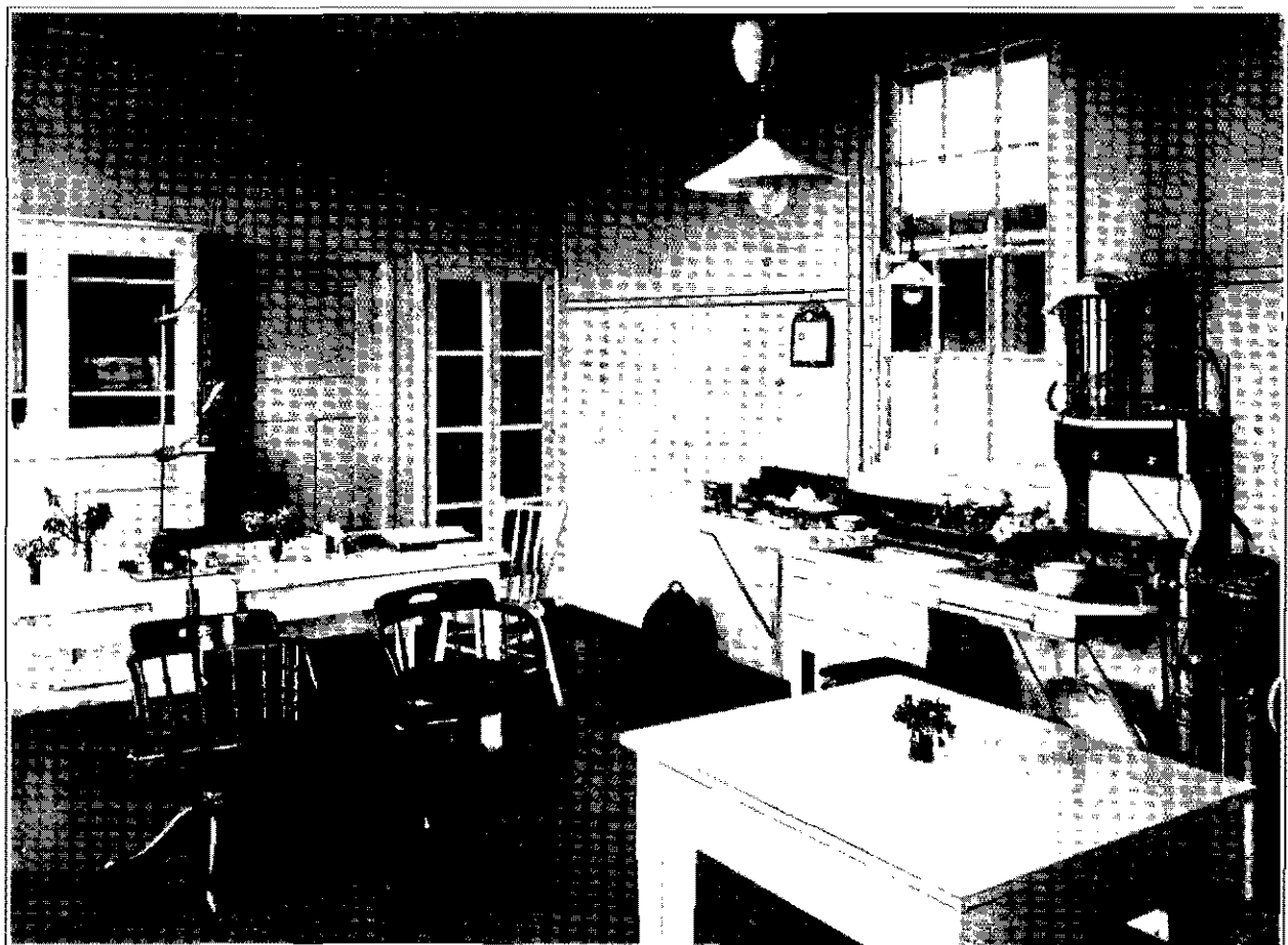
CASUALTY ROOM, NEWPORT WORKSHOPS. (INTERIOR VIEW.) (See page 26.)
